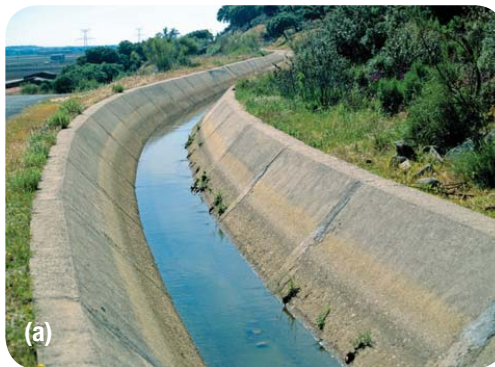
Figure 11 (a) To create a more laminar flow, this waterway is lined with concrete. (b) Concrete baffles help release some of the water's energy by creating more turbulent flow.
